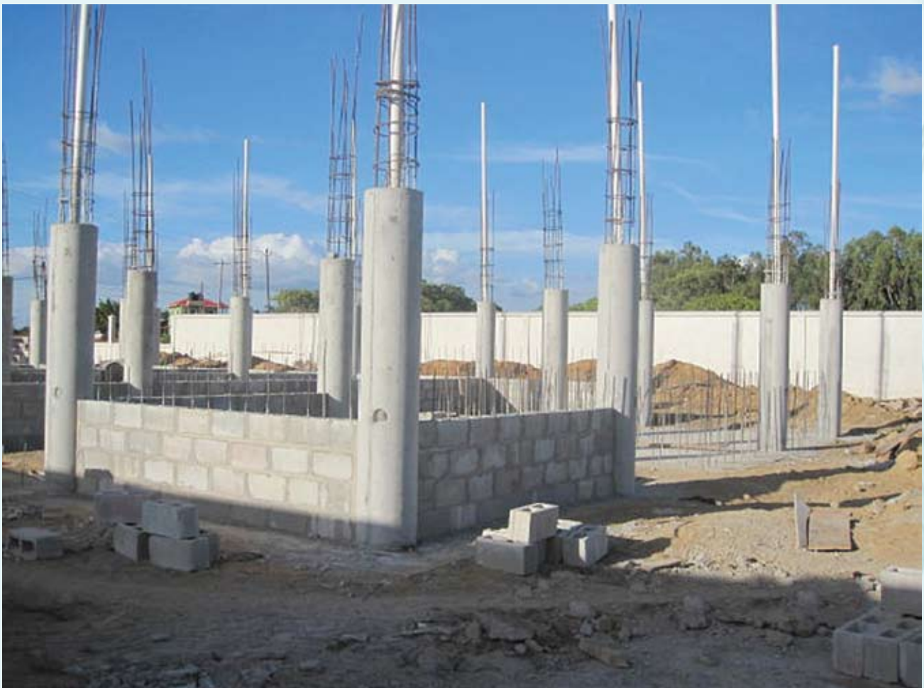
Construction of Lethem Branch Building in progress
